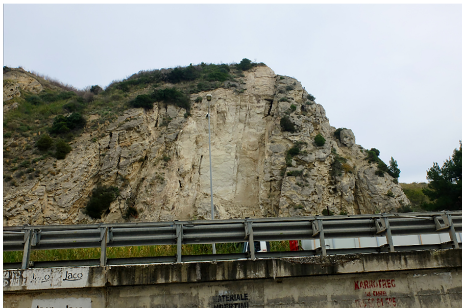
Figure 14. Rock slide aside the road SH4 southward from Durres. Despite occurred after the heavy rains that followed the earthquake, presumably, it was triggered by seismic shaking. Site 2 of Fig. 8.
