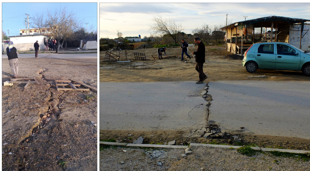
Figure 15. Ground fracture near the water pumping station of Hamallaj (site 12 of Fig. 8).
