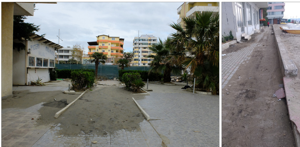
Figure 10. Liquefaction contributed to damage some buildings along the beach of Durres (site 3 of Fig. 8).
