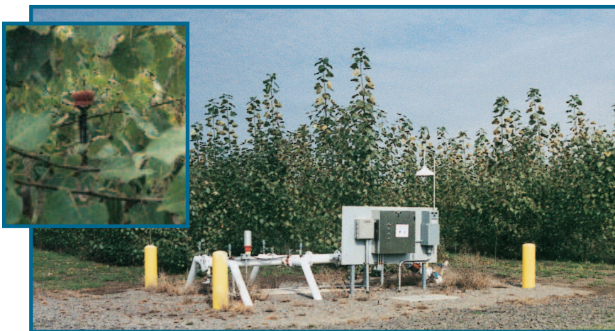
When irrigated with municipal and industrial effluent, hybrid poplar stands have proved highly effective in wastewater treatment and water quality improvement. Shown here is a wastewater pumping station and a closeup of an irrigation stake.
