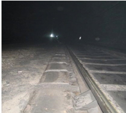
Fig. 8. After the removal of coal dust from the tunnel
