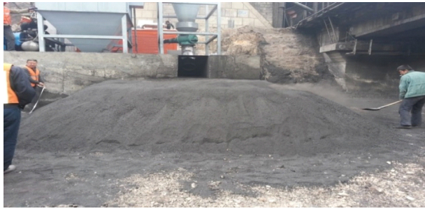
Fig. 6. Coal-dust removal in the Zhangjiawan tunnel
