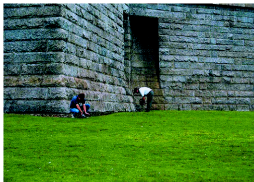
Fig. 12. In the Statue of Liberty National Monument, in-ground Sentricon stations were installed in soil outside the monument walls for a continuing monitoring and early detection of new termite infestations.
