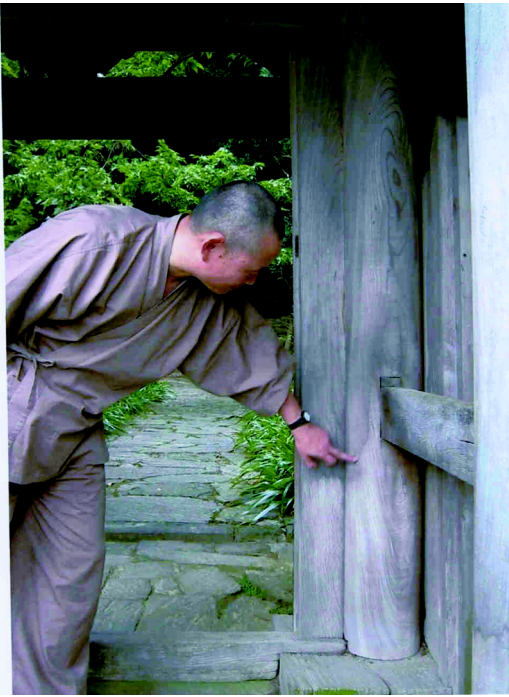
Fig. 10. A Jushoku (resident monk) of a Buddhist temple, Cho-ho Ji, points out stain marking on a 500-yr-old gate post caused by insecticide spraying to control Co. formosanus .
