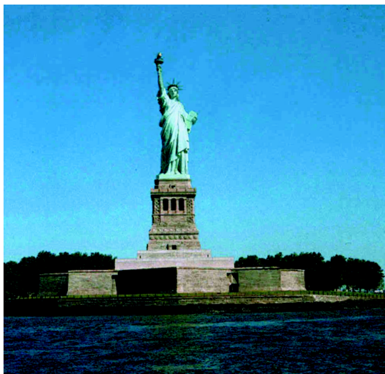
Fig. 9. Many historic structures such as the Statue of Liberty National Monument are located next to harbors, and injecting a large quantity of liquid insecticide in soil may contaminate marine habitats.
